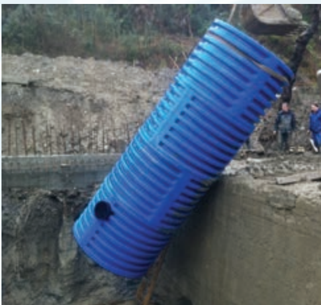
Vertical Pump Stations
